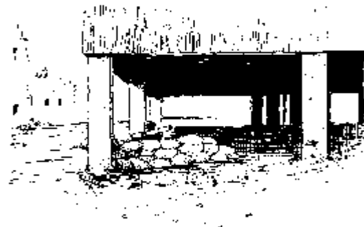
Position with overhead cover
